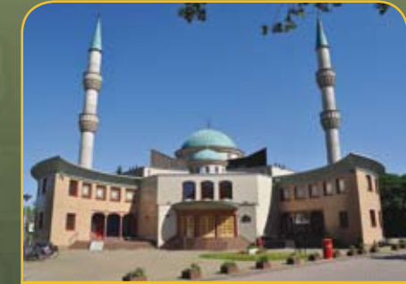
Süleymaniye Camii Tilburg, The Netherlands June 2011
